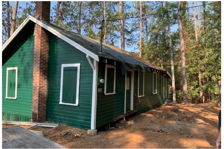
This picture was taken in fall of 2020 after demolition of the shed. This is what the camp looked like when originally built.
