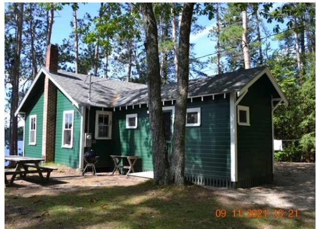
September 2021– Shed 3 is complete.
