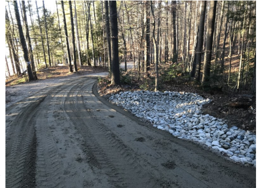
The 23 rd Street Allen Project rocked line ditch and turnout. Grading and compacting of gravel still in progress. Lake is seen on left.
